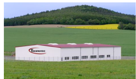
Thermotec production hall
